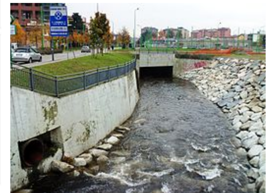
Tunnelling of Seveso River
