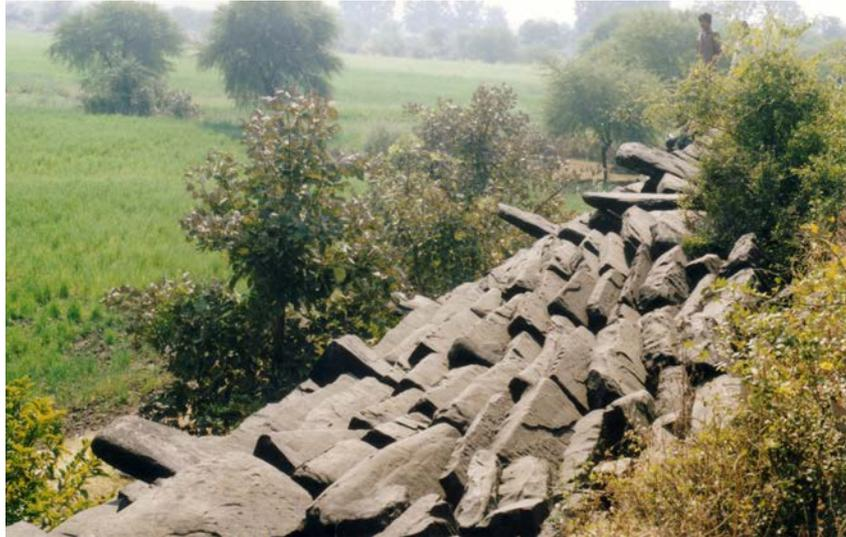
**Plate 8.5** Masonry on the upstream side of the Morel Kala dam, central India.
