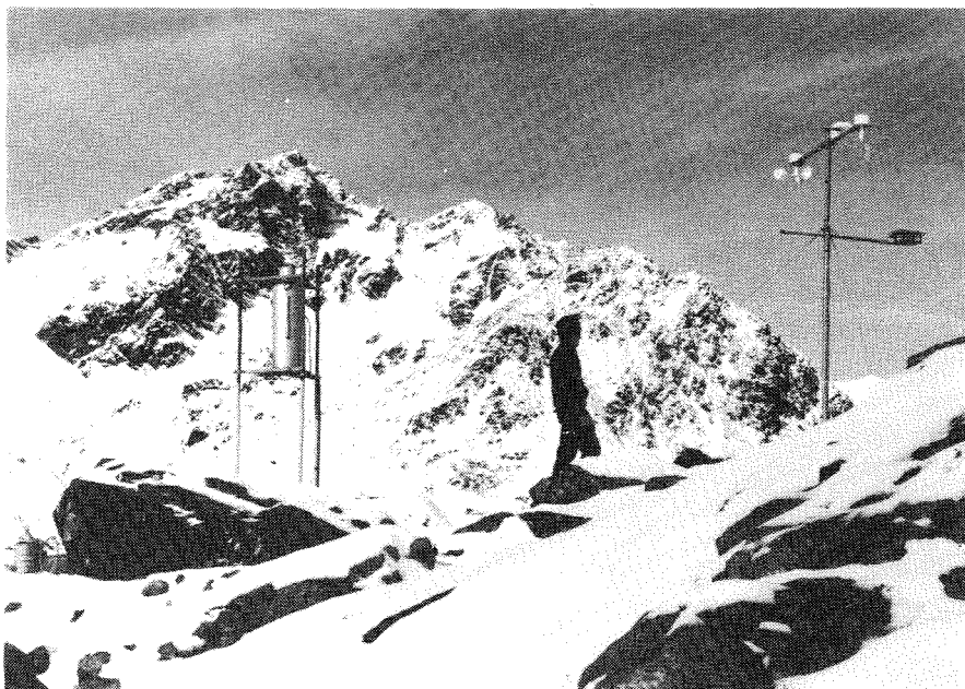
FIGURE 1. Automatic meteorological station (Wallingford-type) operated in the Dischma basin, Swiss Alps, at 2370 m a.s.l. (in 1974). (Photo E. Wengi).
