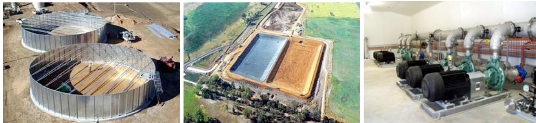
Fig. 4 Wimmera Mallee Pipeline: Left: A typical tank (before lining and roofing). Middle: A typical balancing storage (left lined, right before lining). Right: Pump station.
