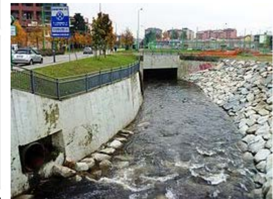
Tunnelling of Seveso River
