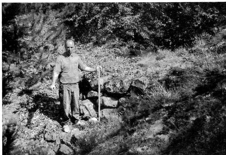
Fig. 4 Check dam of dry laid masonry and afforestation with Austrian pine (Lještarska Dolina drainage basin).
