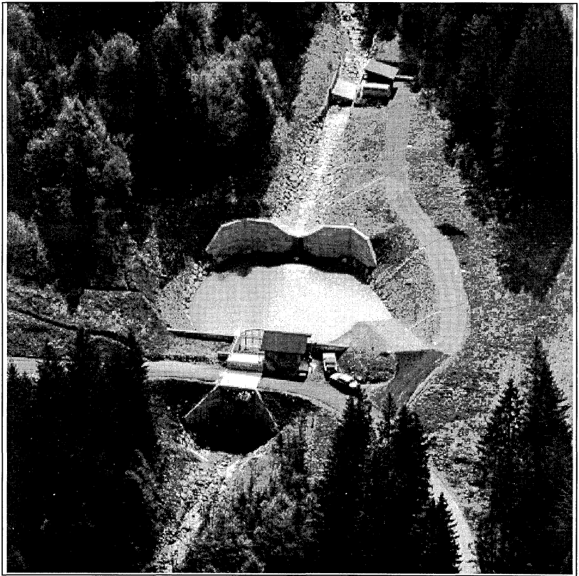
Fig. 1 Sediment retention basin in the Erlenbach stream with a streamgauge. The hydrophone sensors to measure bed load transport are installed at the check dam above the retention basin.
