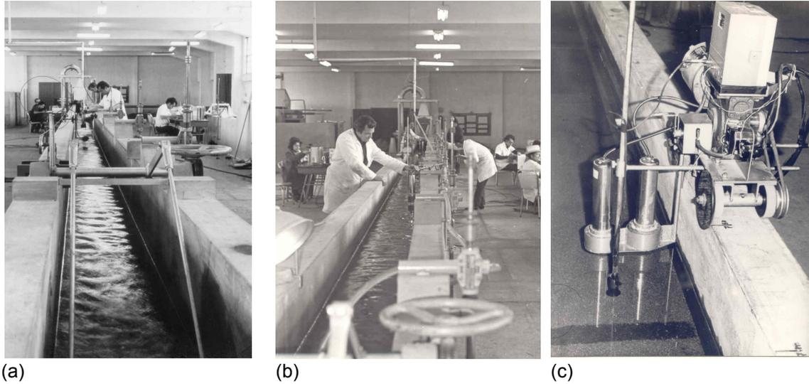
**Fig. 1** (a) The channel at the Institute of Hydraulic Research of the University of Rio Grande do Sul; (b) single grain manual detection system, and (c) labelled particles injected at the mobile bed and automatic detection system.
