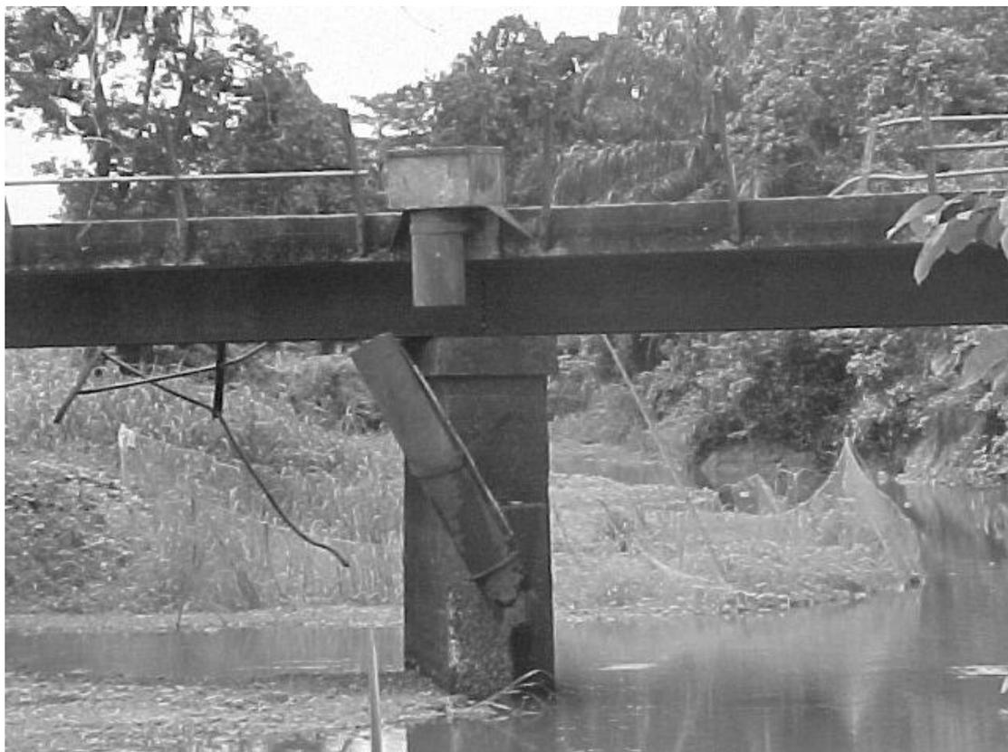
**Fig. 2** Damaged gauging station at Ebute Igboro (Yewa catchment).
