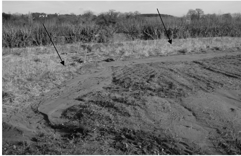
Fig. 2 Sediment deposition at the interface between the buffer and the field at Site 4 due to a “step” between the two created by tillage. The arrows mark the start of the buffer.
