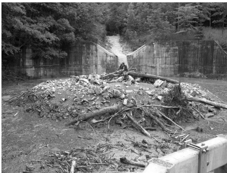
Fig. 1 Debris mound deposited in the retention basin after the flood on 20–21 June 2007 (photo by Patrick Schleppe, WSL Birmensdorf, used with permission).
