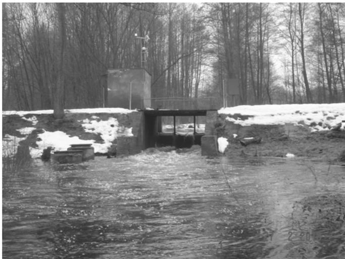
**Fig. 3** View of the stream gauging station at Czarna (photo is looking upstream and was taken at a discharge, which is close to the 2-year flood).
