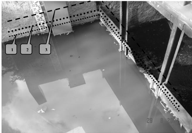
**Fig. 2** Upstream view of the sharp-crested weir of the gauging station at Czarna (the notation 1 indicates the water level at mean discharge, 2 is the water level above which the samples for suspended sediment analysis were taken, and 3 is the water level corresponding to the 2-year flood).
