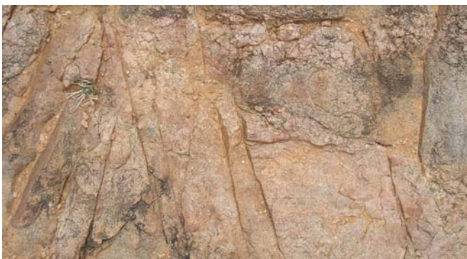
Fig. 2 Fractures seen in a granitic outcrop.
