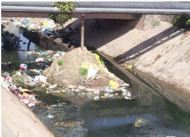
A large mass of silt, waste material and plastic bags accumulated around a small pole in the canal
