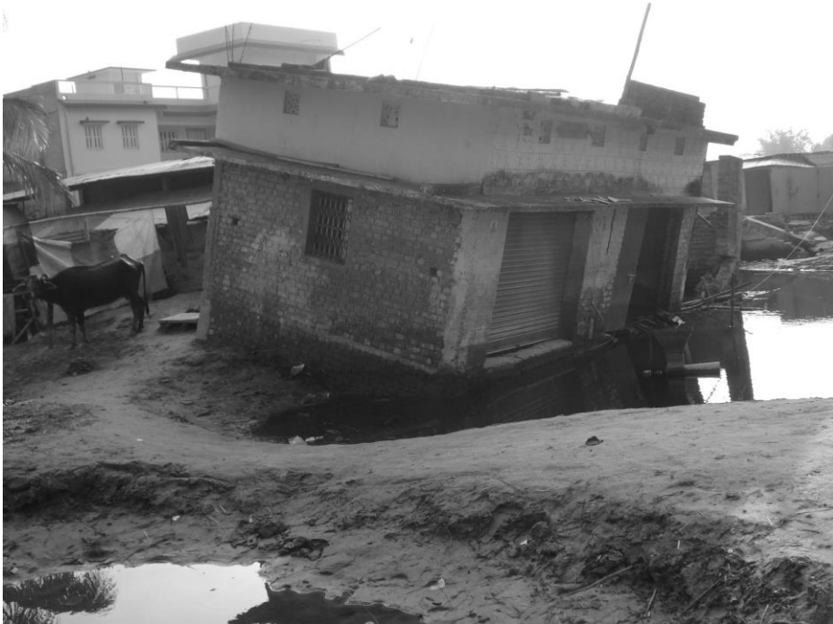
Fig. 3 Damage caused by the Kosi flood in Birpur, Bihar (India).
