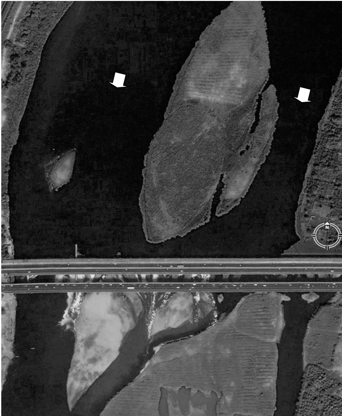
Fig. 2 The barrage near ITO on the River Yamuna, Delhi.
