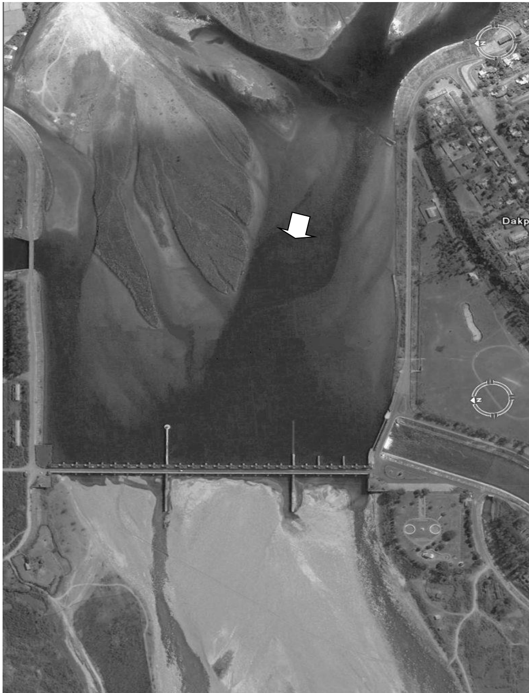
Fig. 4 The Dakpathar barrage on the River Yamuna.
