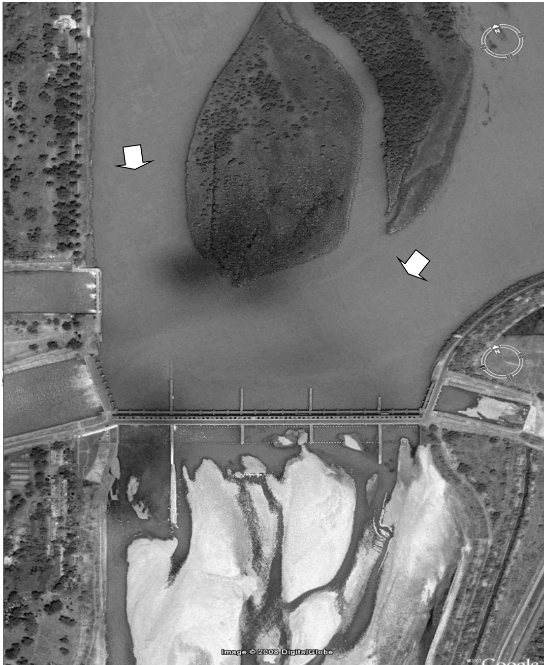
Fig. 6 The Bhimgoda barrage on the River Ganga at Haridwar.
