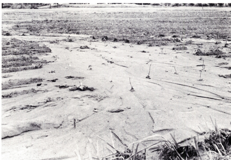
FIG.3 Breaks in improperly constructed terraces can cause severe gullying.
