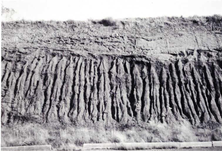
FIG.6 Initiation of serious erosion.
