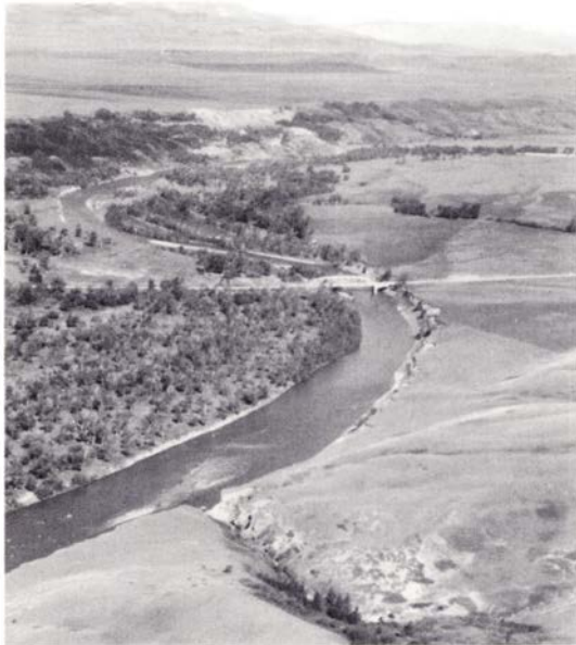
FIG.2 View to northwest across the Oldman River north of the Three Rivers site.
