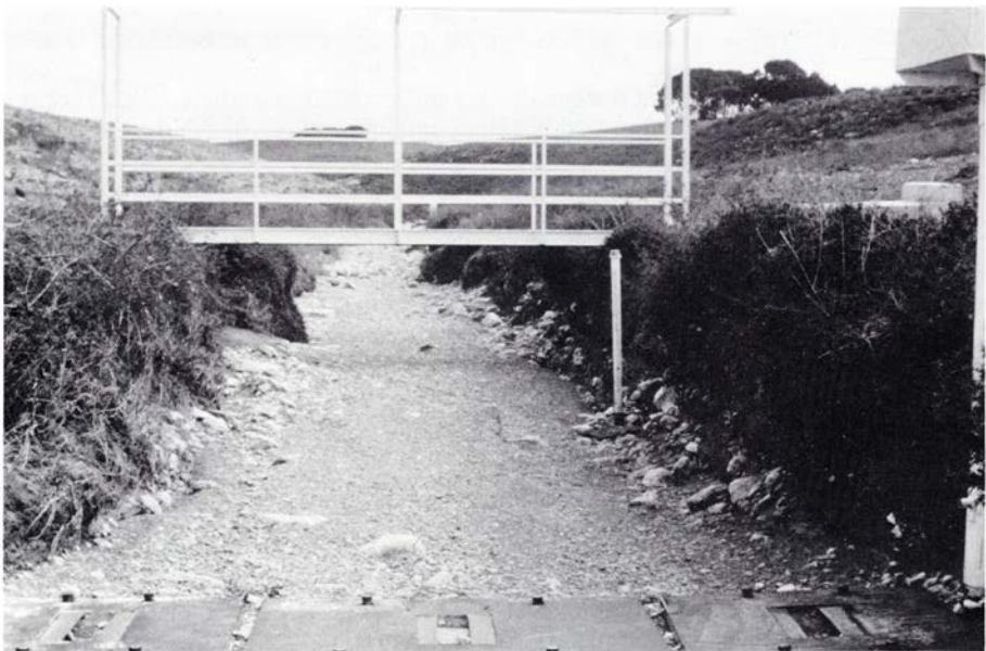
FIG. 3 Sediment transport monitoring station on the Nahal Yatir after a flash flood showing the approach reach and the sampler slots.
