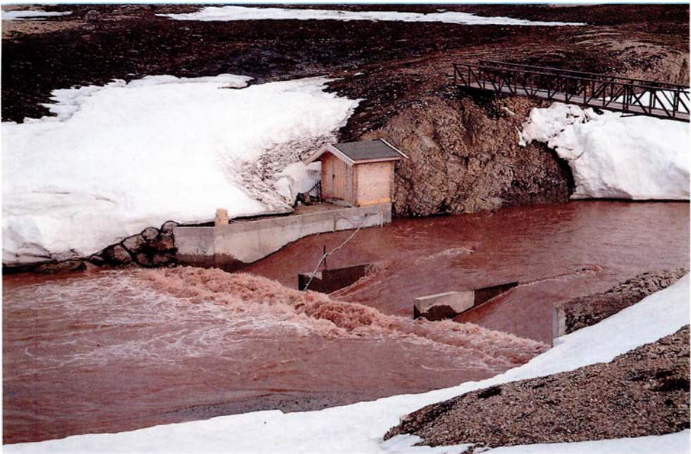
FIG. 2 The monitoring station with the composite crump weir in river Bayelva at Svalbard in the High Arctic.
