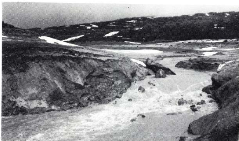
FIG. 7 Erosion of the passage between basins I and II of Målvatna.
