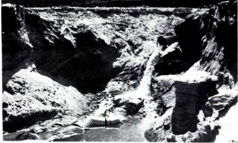
FIG. 1 Creek degradation and unsuccessful repair attempt, Gjevilvannet.
