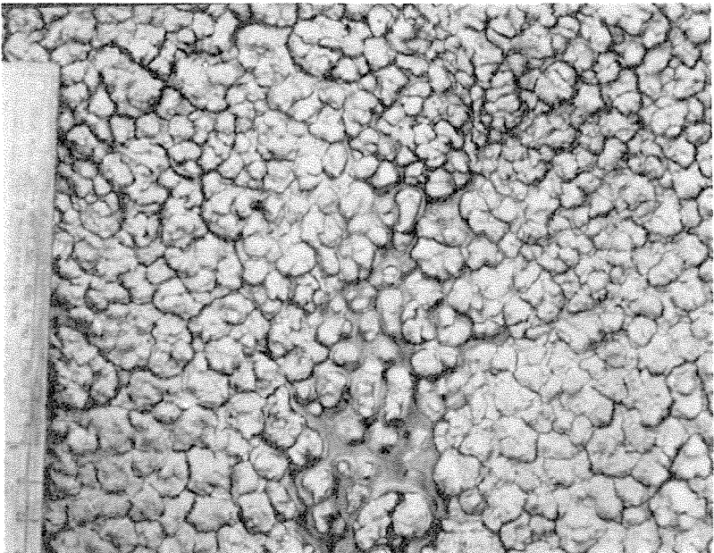
Fig. 2 Initiation of runoff on montmorillonitic shales prior to closing of desiccation cracks.
